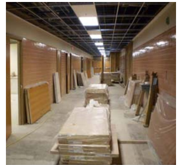
Construction at Sierra Middle School
